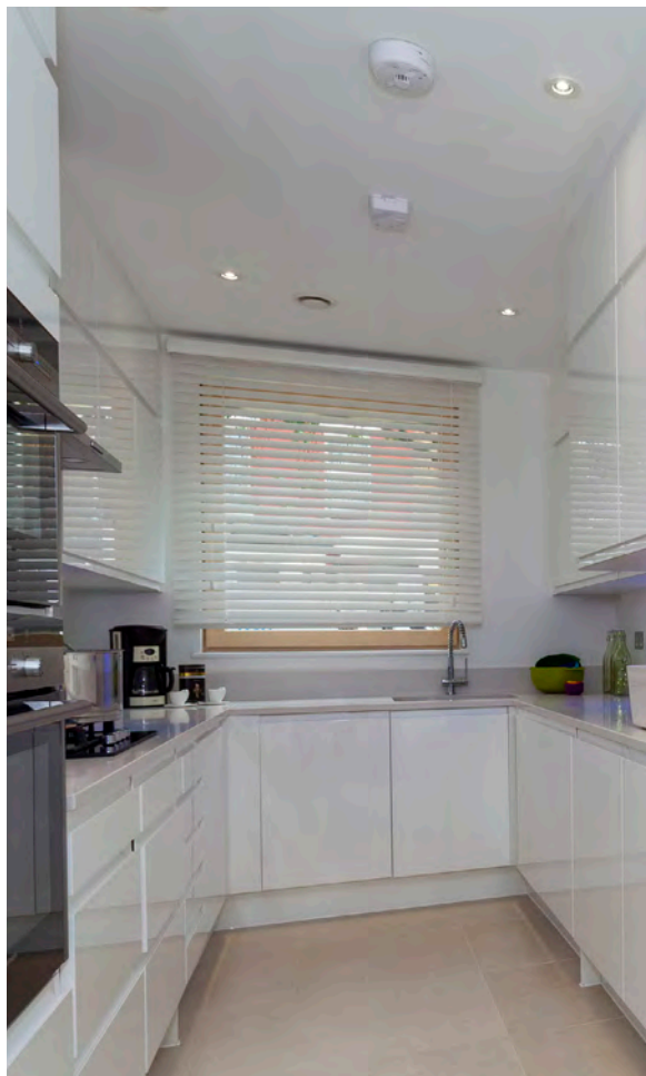
Mechanical ventilation extract
