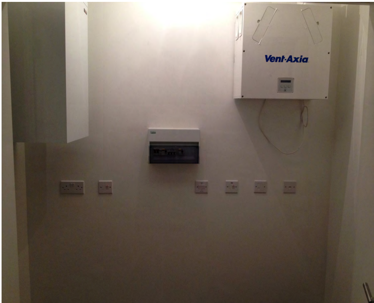
Utility cupboard with a Mechanical Ventilation and Heat Recovery unit (MVHR), distribution unit and washing machine space
