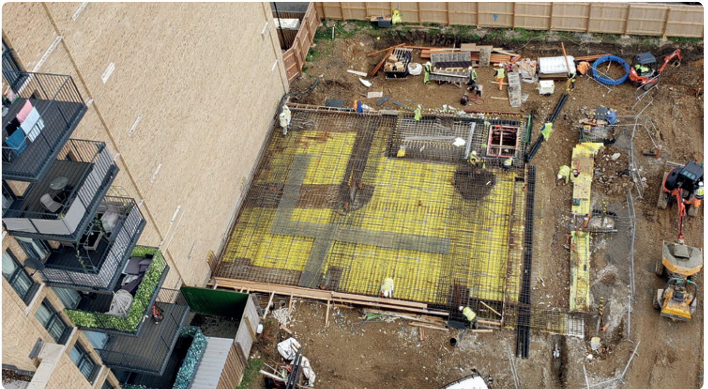
An aerial view of Phase two Sherwood Close which is underway
